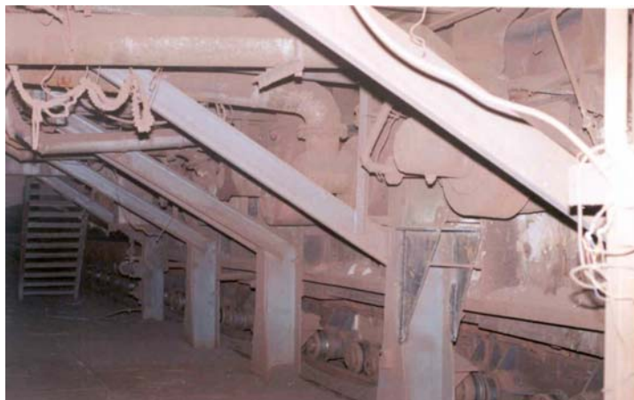
Figure 1. View of the sinter furnace before modification
