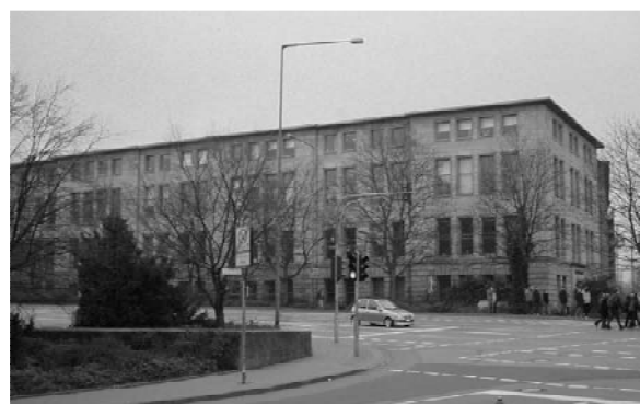
Fig. 12 Institute of Ferrous Metallurgy, today
