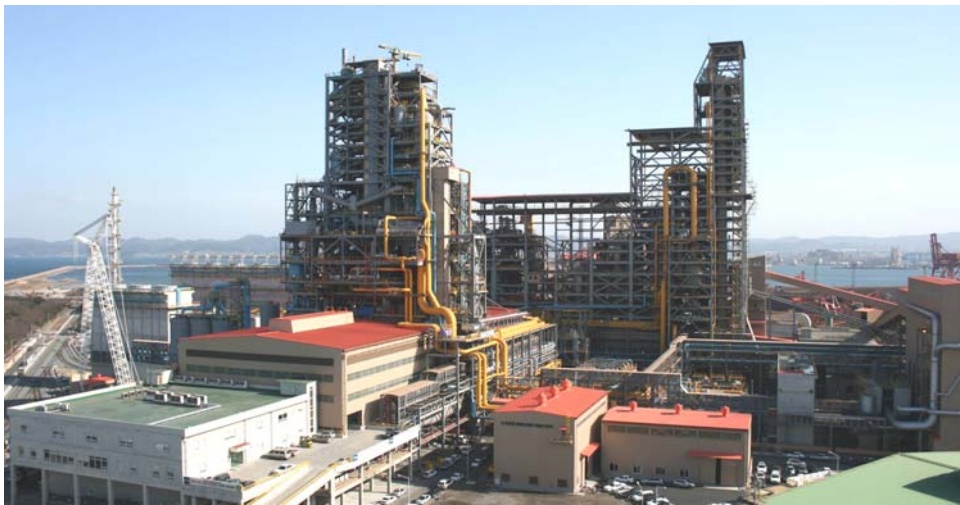
Figure 14: FINEX 1.5M Plant at the Pohang Works
