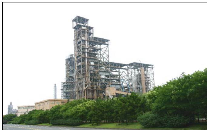
Figure 7: FINEX Demonstration Plant, Pohang Works, Korea
