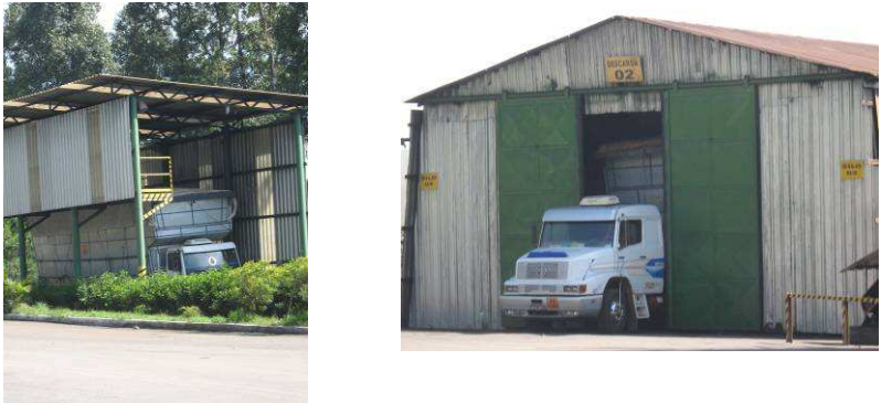
Manual volume measurement of loose coal - Brazil
