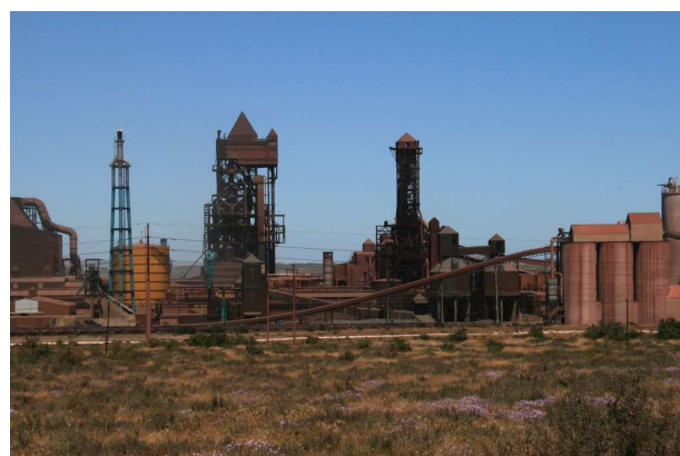
Figure 8: COREX C-2000 DR combination Saldanha.
